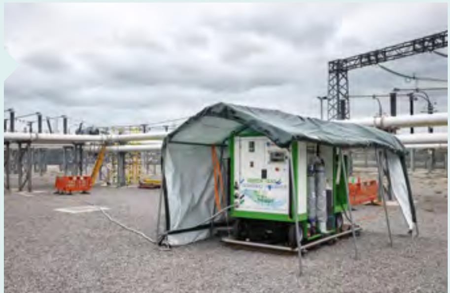
Onsite gas cart used to retro fill existing gas-insulated, high-voltage switchgear, with an alternative low global warming g<sup>3</sup> gas, designed for high-voltage transmission equipment, Richborough Substation, Kent, UK
